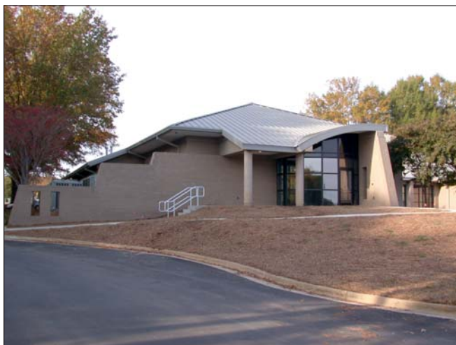
I.T. BUILDING WITH STANDING SEAM ROOF
