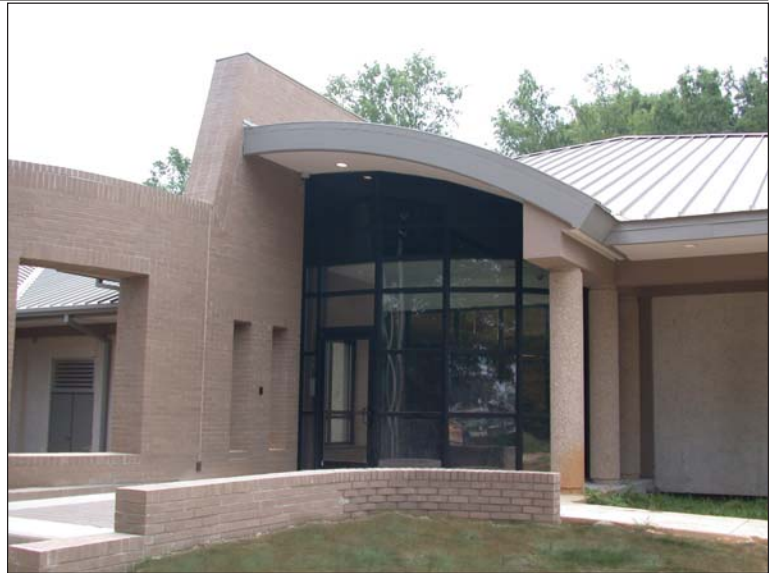
SECURITY FINANCE BUILDING FEATURES RETROFIT METAL STANDING SEAM ROOF
